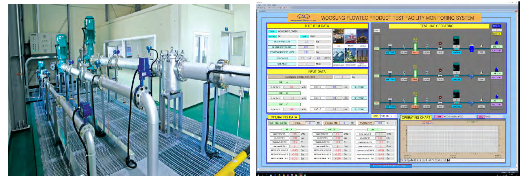
Pressure drop test
